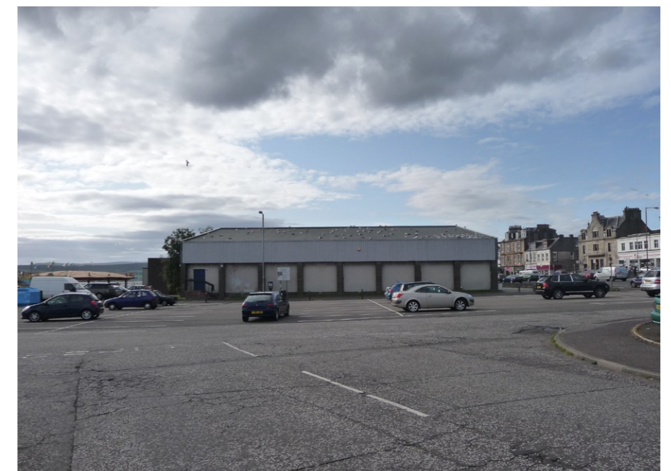
3.2 Existing pool building from the east
