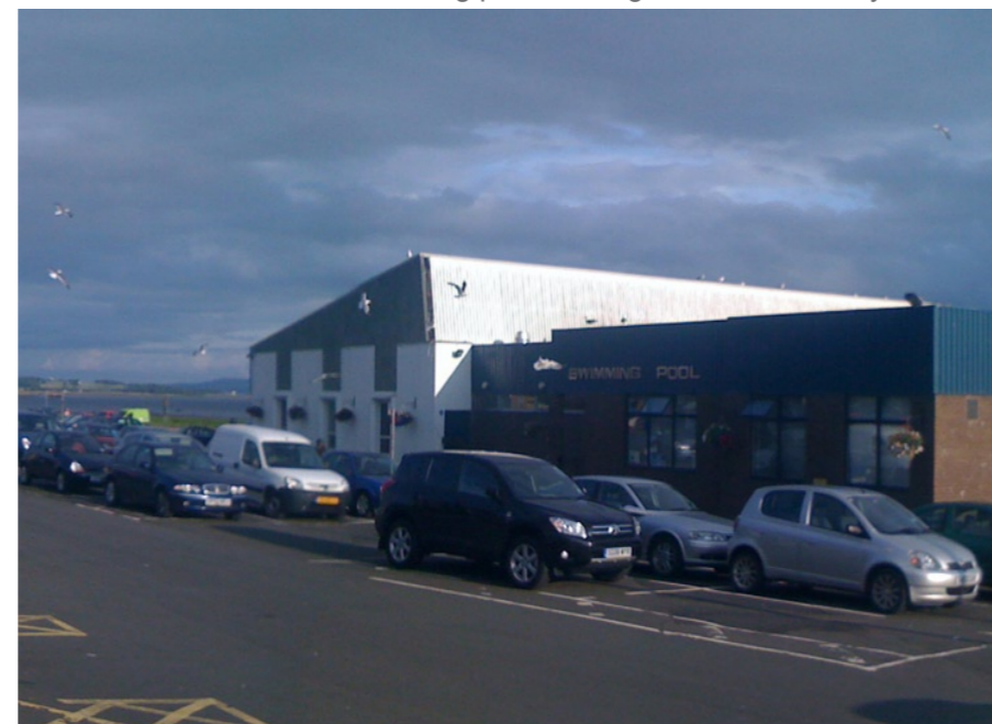
3.2 Existing pool building from the West Clyde Street
