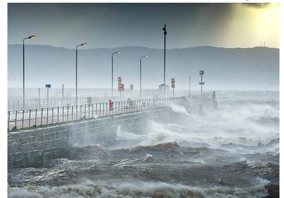
3.3 Pierhead during storm
